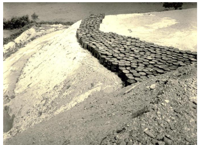
Figure 3: Constitution of a drum layer.
